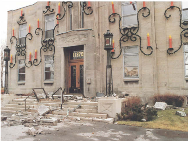
Figure 7. Magnitude 5.9, Saguenay, Quebec, 1988. Masonry damage to the former Montréal East city hall. More than 300 kilometres from the epicentre, this structure is founded on 17 metres of clay which amplified the earthquake vibrations
