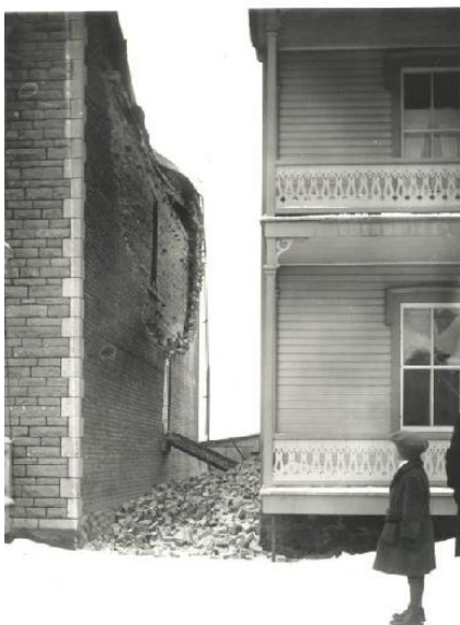
Figure 2. Damage to brick wall in Shawinigan, Quebec, more than 200 kilometres from the epicentre of a magnitude 6.2 earthquake, Charlevoix, Quebec, 1925 Source: Photo from Lamontagne, M. and Bruneau, M. 1993
