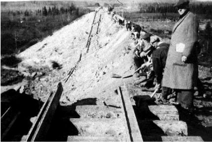
Figure 4. Magnitude 6.2, Témiscaming, Quebec, 1935. Some 300 kilometres away from the epicentre, near Parent, Quebec, vibrations from this earthquake triggered a 30 metre slide of a railroad embankment
