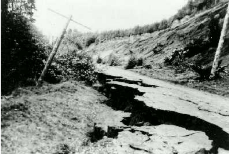
Figure 6. Magnitude 7.3, Vancouver Island, 1946. Soil Failure on the Kelsey Bay Highway, north of Campbell River, British Columbia
