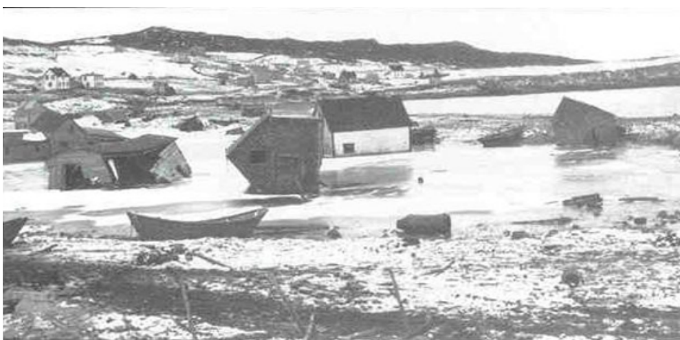
Figure 3. Magnitude 7.2, Laurentian slope, offshore Newfoundland, 1929. Buildings in Lords Cove, Newfoundland tossed and smashed by the tsunami Source: Photograph by H.M. Mosdell, from the collection of W.M. Chisholm; published in GSC Bulletin 548 "A Synthesis of Geological Hazards in Canada" G.R. Brooks, Editor
