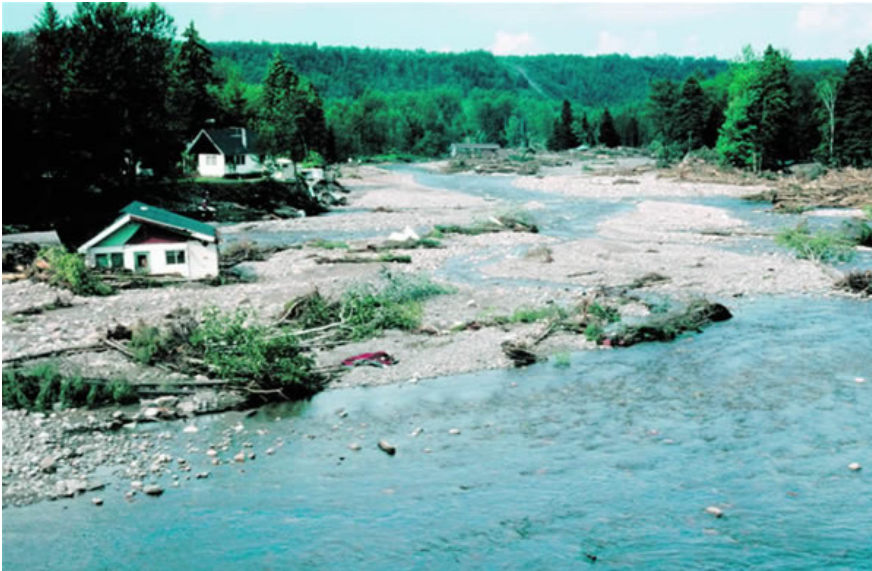
Figure 4. Photograph of a house washed off its foundation and located on a river channel after the flood, Saguenay area, July 1996
