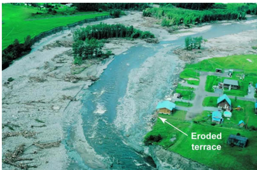
Figure 5. Photograph of buildings on a terrace undermined by bank erosion, Saguenay area, July 1996
