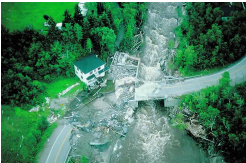
Figure 6. Photograph of a bridge crossing where the constriction formed by the bridge abutments has caused floodwaters to spill over the bridge, Saguenay area, July 1996
